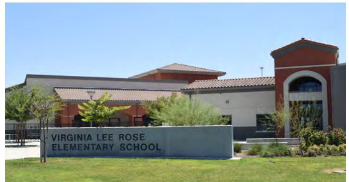
Virginia Lee Rose Elementary School, Madera Unified School District
