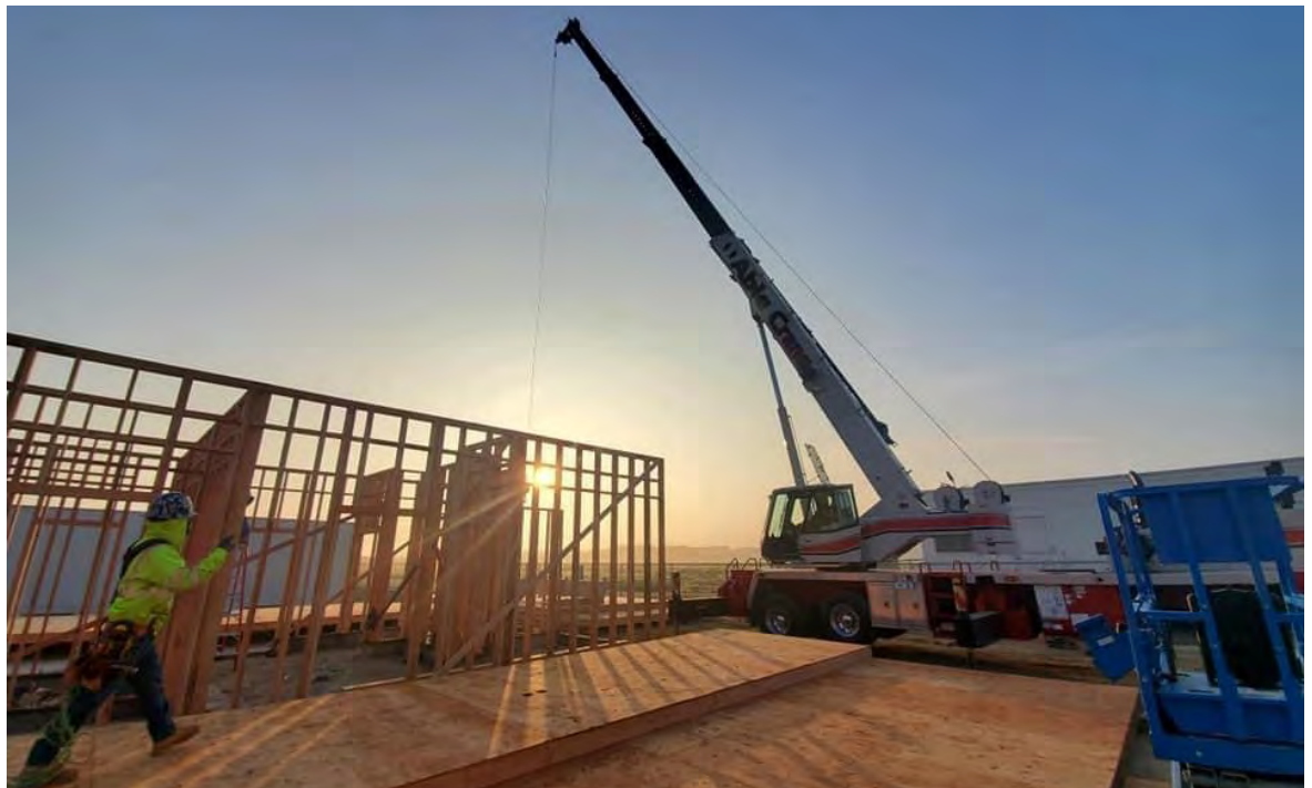
Bush Construction: Liberty Elementary School Kindergarten Addition, Liberty Elementary School District
